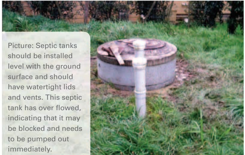
Picture: Septic tanks should be installed level with the ground surface and should have watertight lids and vents. This septic tank has over flowed, indicating that it may be blocked and needs to be pumped out immediately.
